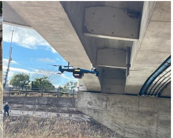
Skydio 2 + flying for inspection of floorboards and support
