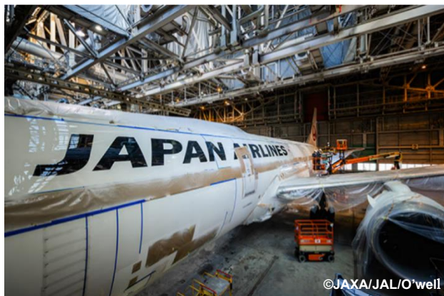
Riblet Application Work Scene
