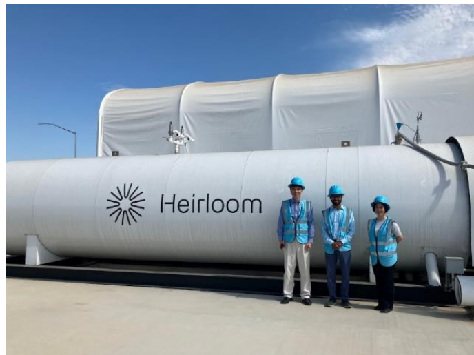
Tanks to store collected CO2
